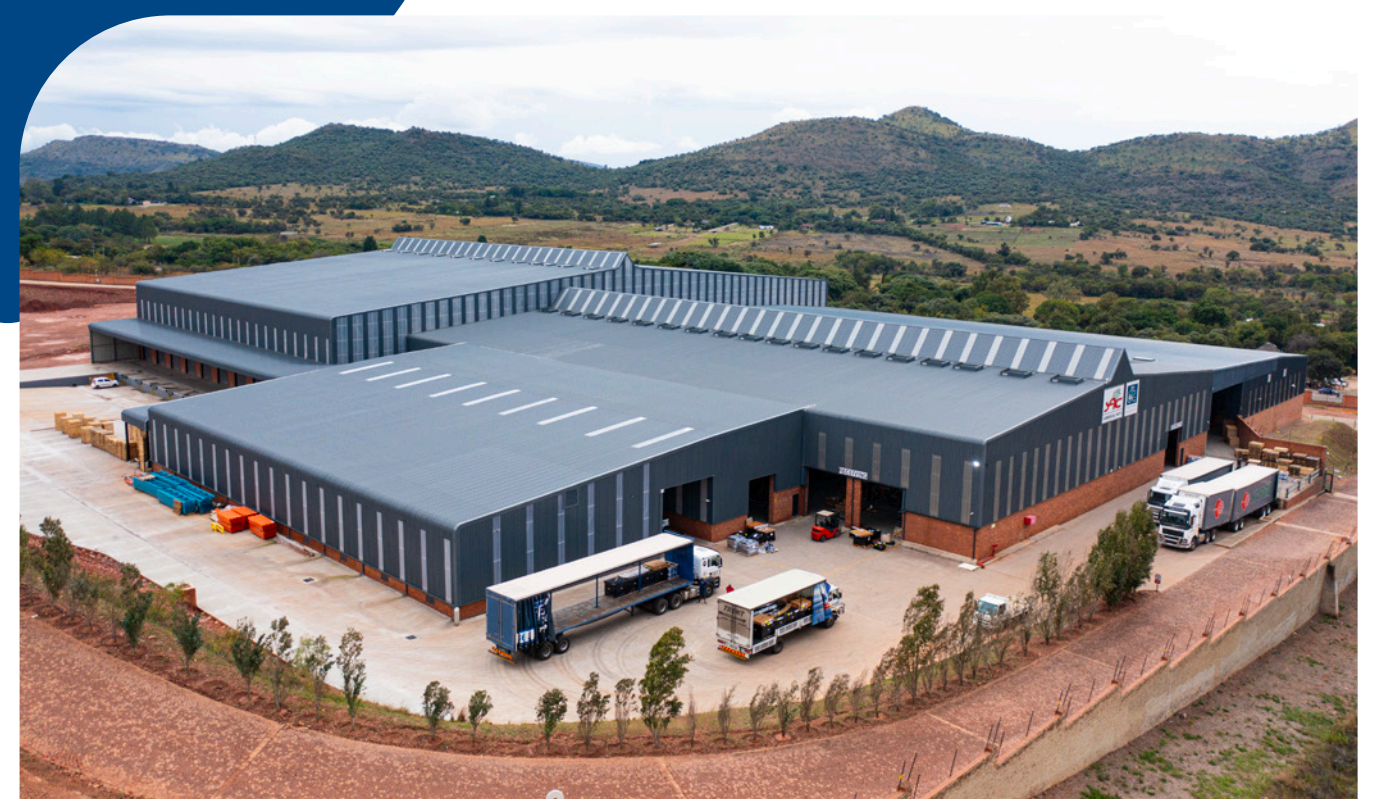
The SAC Commercial Parts central warehouse, opened in 2019, is located in Centurion between Pretoria and Johannesburg.
