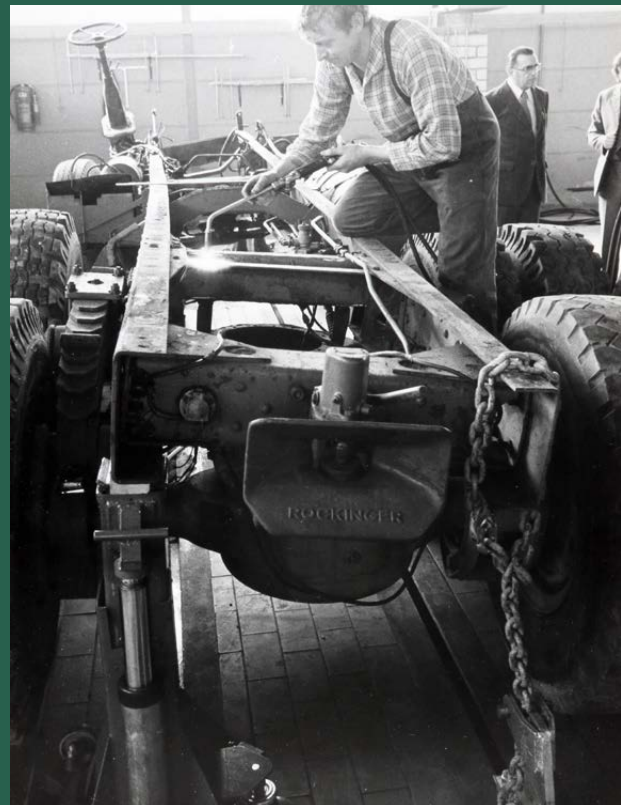
In 1972, the Knirsch workshop in Karlsruhe is equipped with the first Josam frame levelling bench in Germany.
