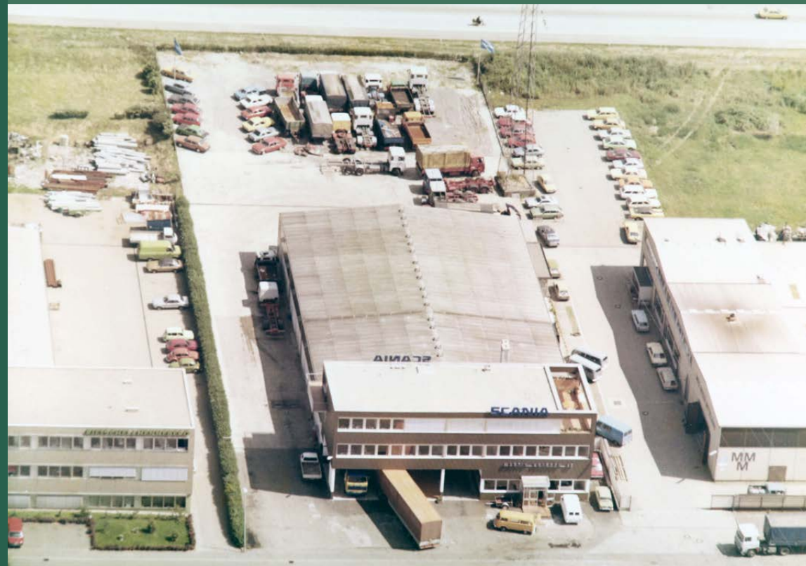
An aerial photograph from 1980 points to the newly expanded workshop of Martin Knirsch Kraftfahrzeuge in Karlsruhe on Ohmstraße.
